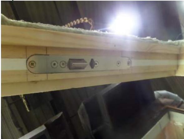
Top latch forend in frame head – doorset A
